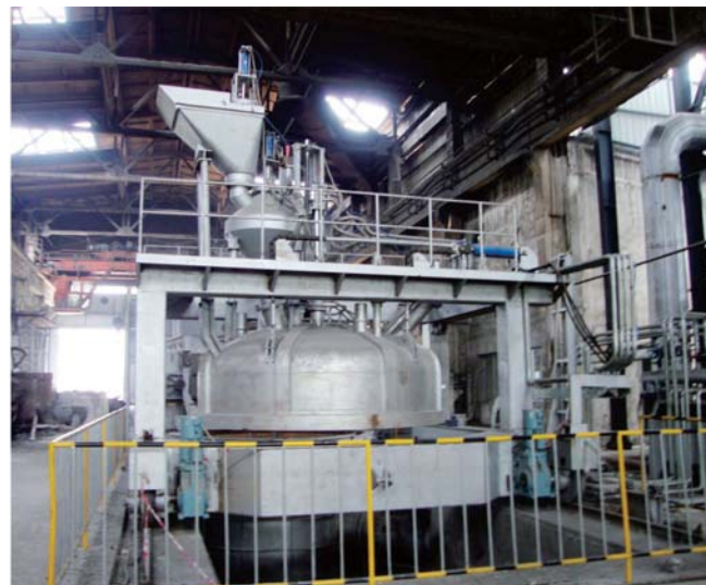
30吨VOD炉 30t VOD Furnace
